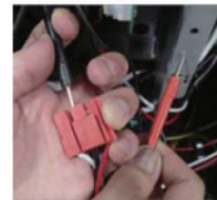
Measuring insulation resistance between fan terminal & chassis
