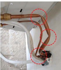
Check Pipe state
