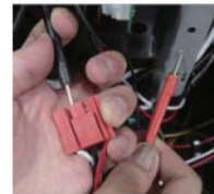
Measuring insulation resistance between fan terminal & chassis
