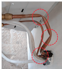
Check Pipe state
