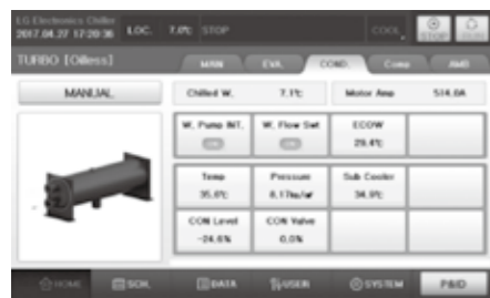
State of condenser
